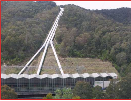
#1 Power Station, Snowy River Scheme
